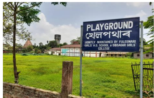
PLAYGROUND UNDER RENOVATION
